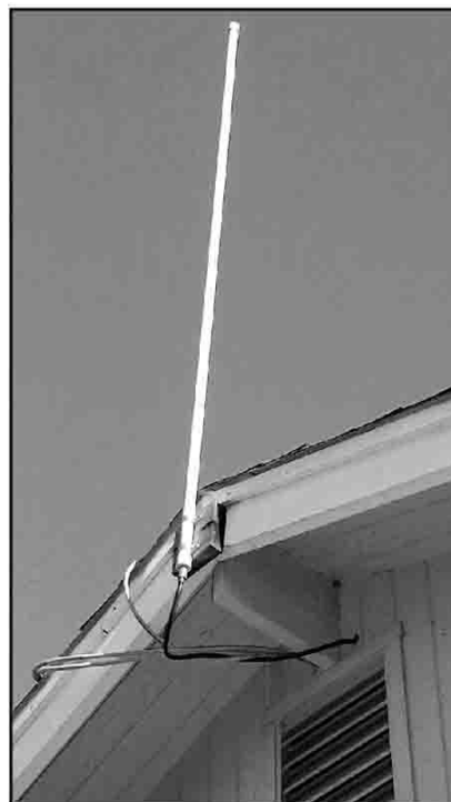
Figure 5—The completed antenna mounted to the roof.
